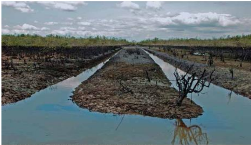
A right of way more than 30 metres wide cut through mangroves
